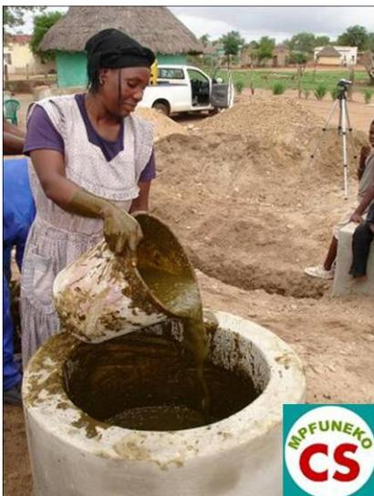
To make sure that the digester produces the amount of gas that the plant is supposed to produce, it is absolutely important to fill the digester properly. To give an idea what it means to fill a 15 cubic meter digester (which produces sufficient gas for three families), it is useful to have a look at the amount of material needed. For a 15 cubic meter digester six 20 liter buckets of cow dung are mixed with six buckets of water. 20 liter of cow dung is about the amount one cow produces per day.
